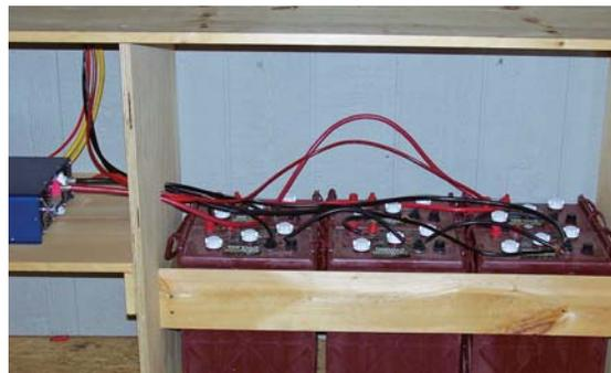
Inside the shed, a bank of six deep-cycle batteries — wired in parallel and in series — receives a continuous charge from solar roof panels and a site-assembled wind turbine.
